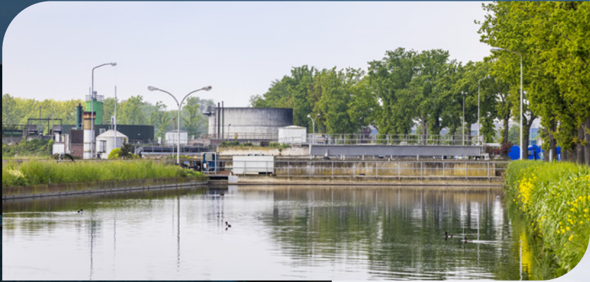
Water treatment facility Lieshout
